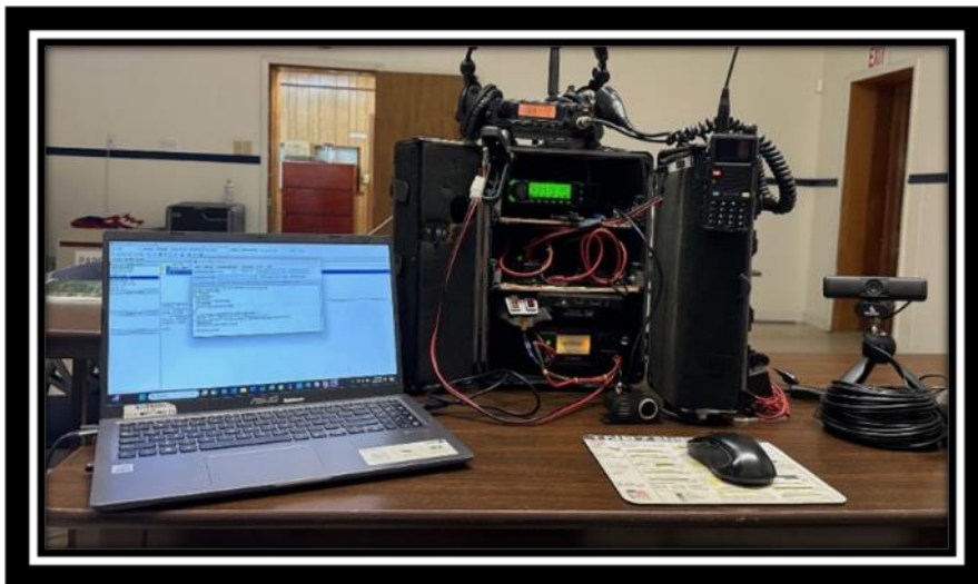
My Station. Battery box on the floor
